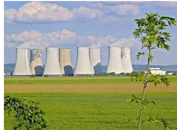
Nuclear Power Plant Bohunice
